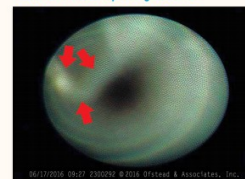
Photo 3. Filamentous debris protruding into channel
